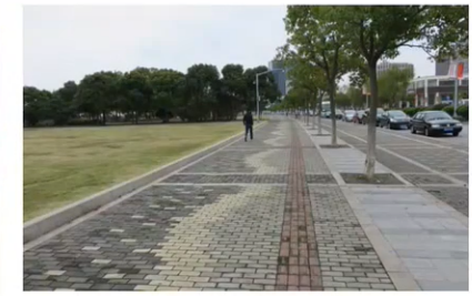
Figure 4 Permeable pavements in Lingang ( https://www.theguardian.com/world/2017/dec/28/chinas-sponge-cities-are-turning-streets-green-to-combat-flooding )
